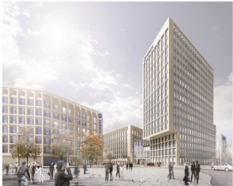
Moving in: Zurich Insurance will centralise its operations into the new MesseCity Köln office district
